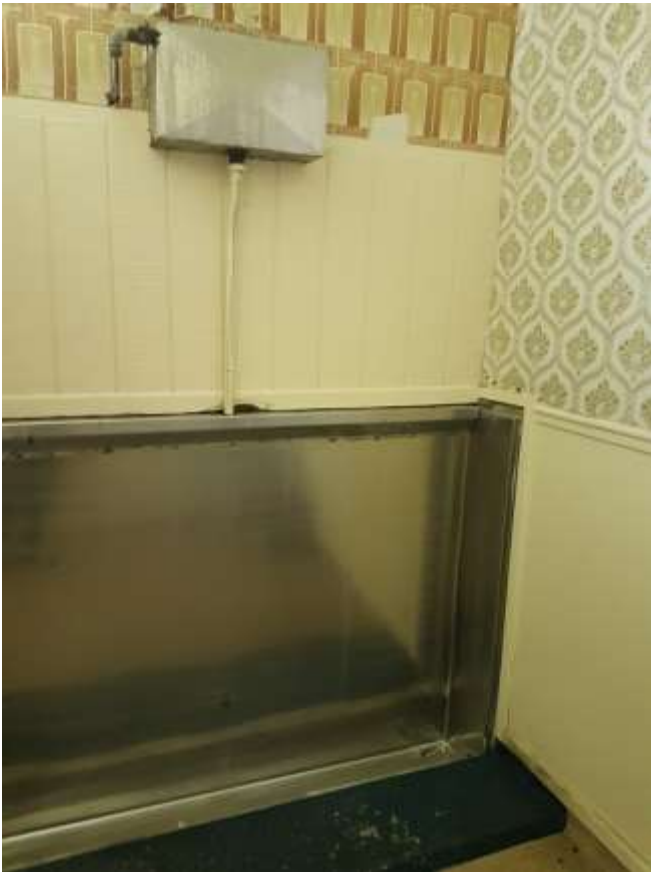
Toilets: The toilets are dated but tidy. However there is some rotten Gib board above the Urinal cistern, and wallpaper coming away in some areas.
