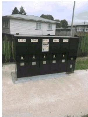
This is a typical high voltage switch that will be used The size of the proposed Halo RMU is 730mm deep X 2400mm long X 1250mm high.
