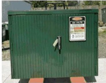
The cabinet shown here is a typical LV cabinet which will replace the Tin sheds The typical size of the cabinets is 1150mm wide x 350 mm deep X 1100mm high.
