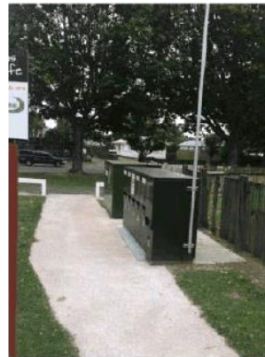
This is a typical high voltage switch that will be used The size of the proposed Halo RMU is 730mm deep X 2400mm long X 1250mm high.
