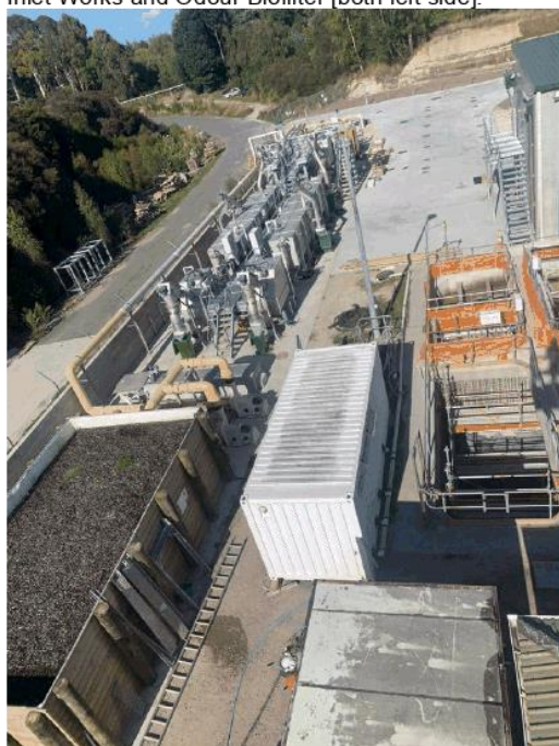
Inlet Works and Odour Biofilter [both left side].
