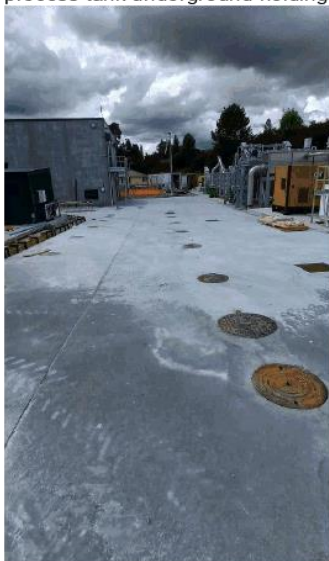
Concrete surfaces poured over process tank underground holding tanks
