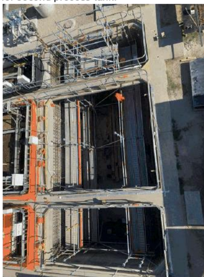
Structural strengthen work underway for second process tank.
