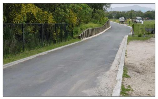
Figure 19: New short/narrow streets like Sherwood Way have tighter curves and pedestrians walking in the street, hence may have low operating speeds and be "self-explaining" at 40 km/h or less
