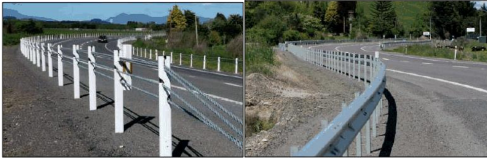
Figure 7 Flexible road safety barrier and guardrail on rural roads (Waka Kotahi)
