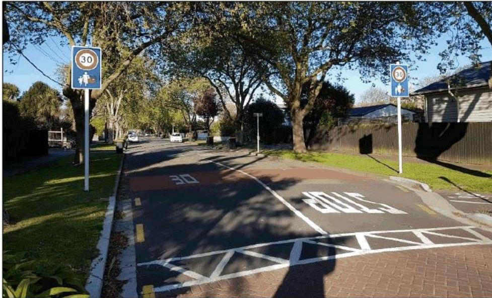
*Figure 3 Low speed street with raised platform and markings*
