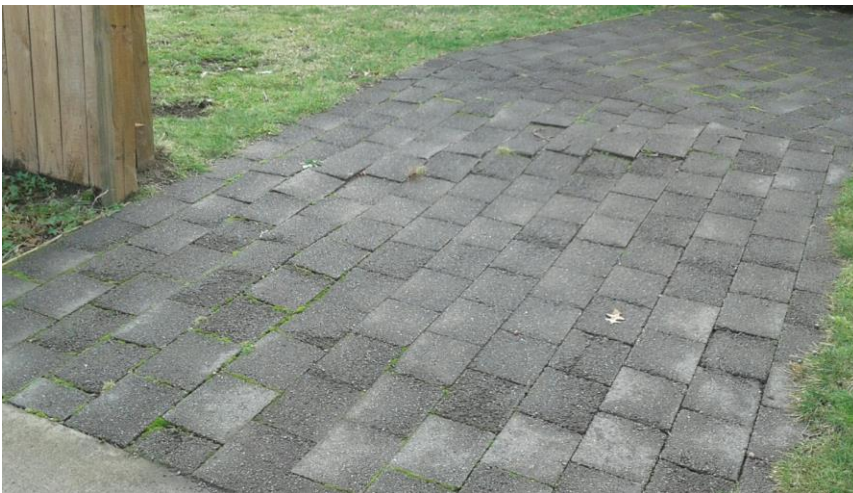
Photograph of root lifting of cobbled driveway.
