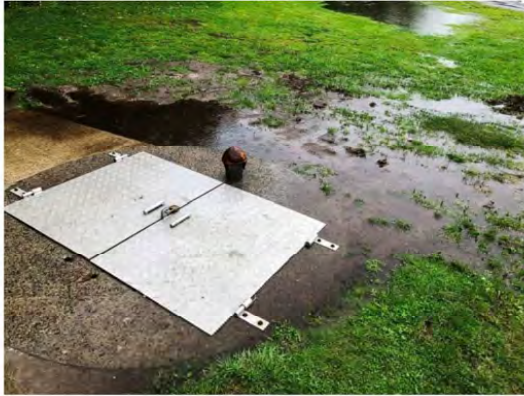
Sewer pump chamber lid with storm water flowing over
