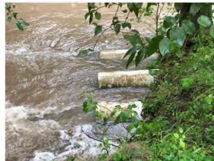
Photo 4. Outlet pipes to stream with lake level at 357.5masl, (lake full) with moderate waves
