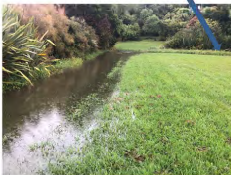
Photo 5. Water ponds along the eastern edge of playing field and will not drain away
