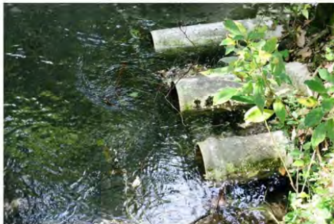
Photo 3. Outlet pipes to stream with lake level at 356.04masl, with small waves
