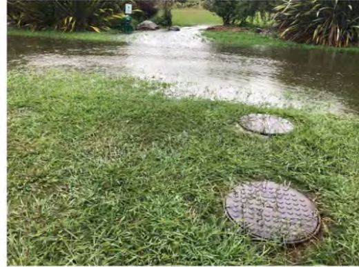
Manholes at end of additional storage pipes. Water was flowing into them before the picture was taken
