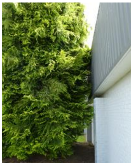
Proximity of trees to building.
