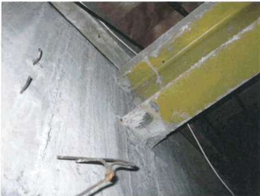
Strongroom at First Floor - Embedded Steel Beam
