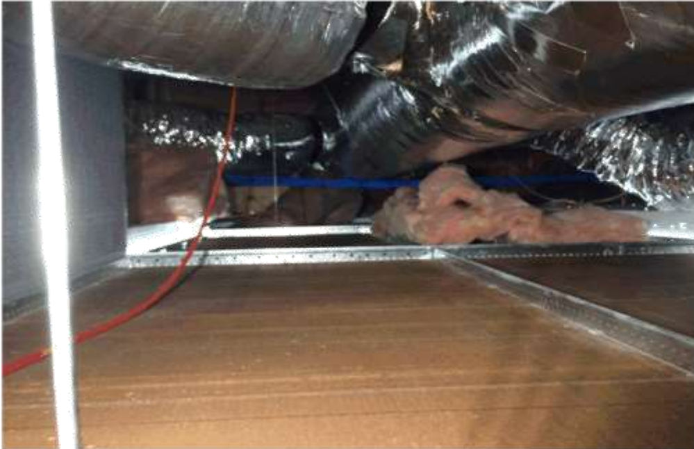
The insulation has been removed in mainly parts of the ceiling tiles.
