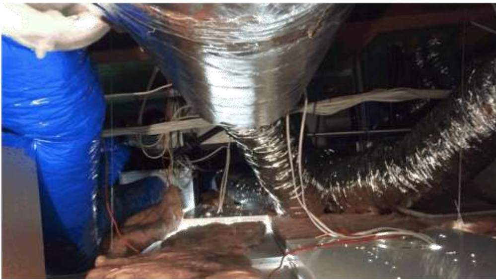
Redundant ducting and loose wiring can cause a fire hazard.
