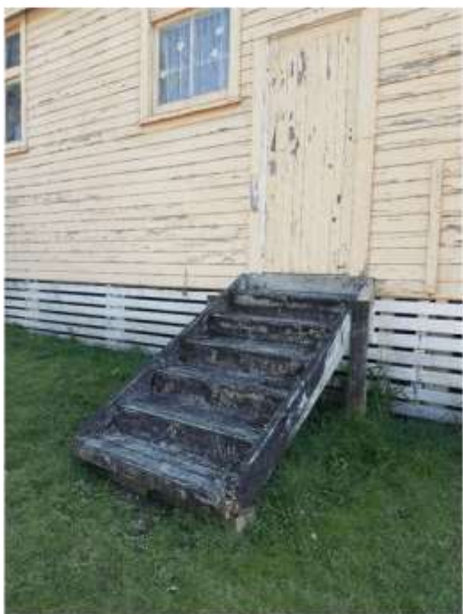
The Emergency exits lead out the back of the building down steps which do not have any handrails installed.
