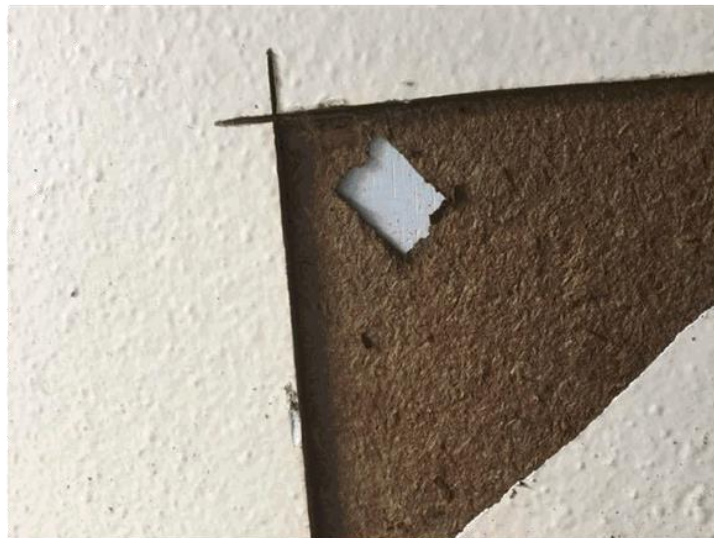
Zone 5 - Insulating Board Secondary Wall Linings - Confirmed ACM
