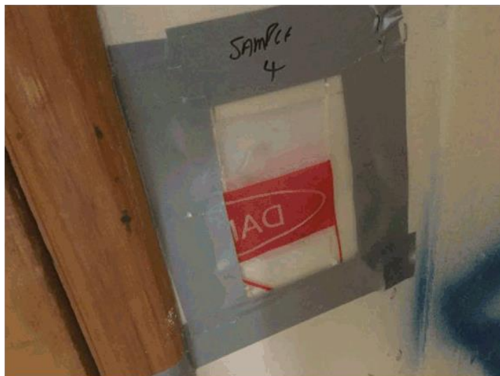
Zone 4- Insulating Board Secondary Wall Linings - Confirmed ACM
