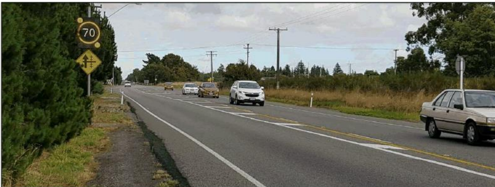
Figure 9 Rural intersection activated warning signs (RIAWS)
