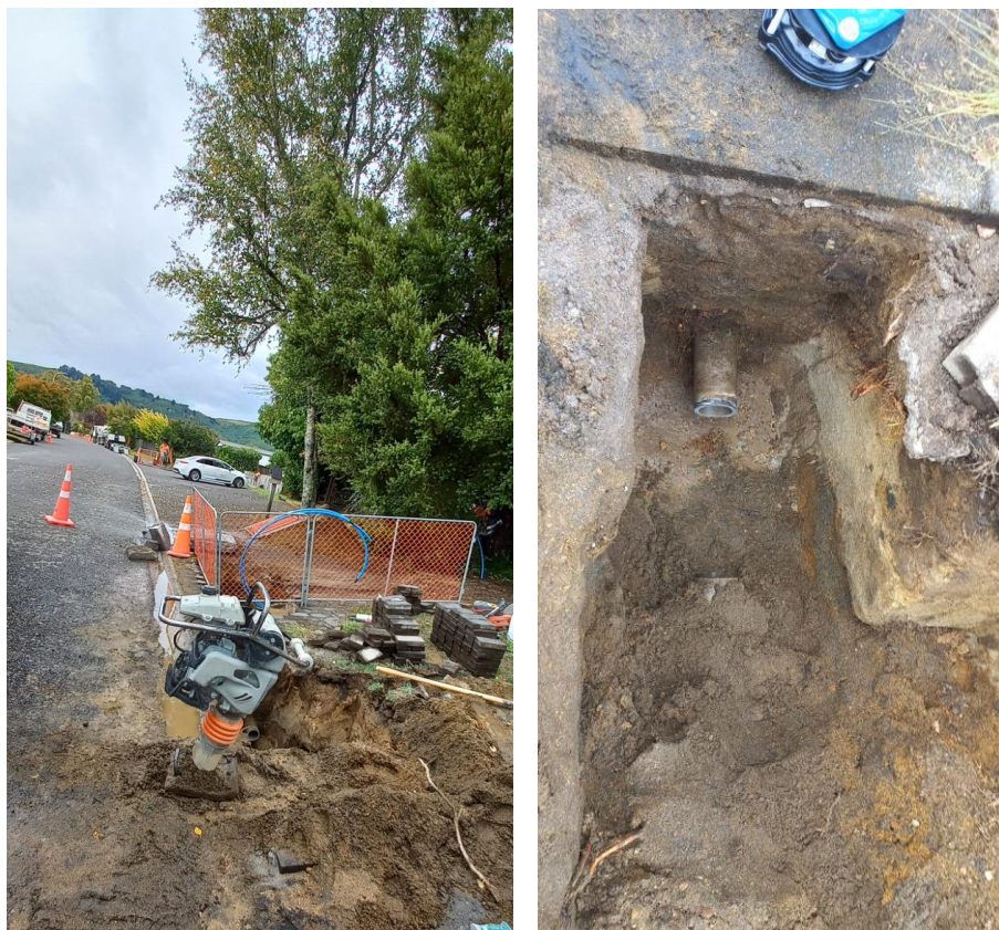
Photographs showing proximity of water line work to trees and minor roots encountered within trench.
