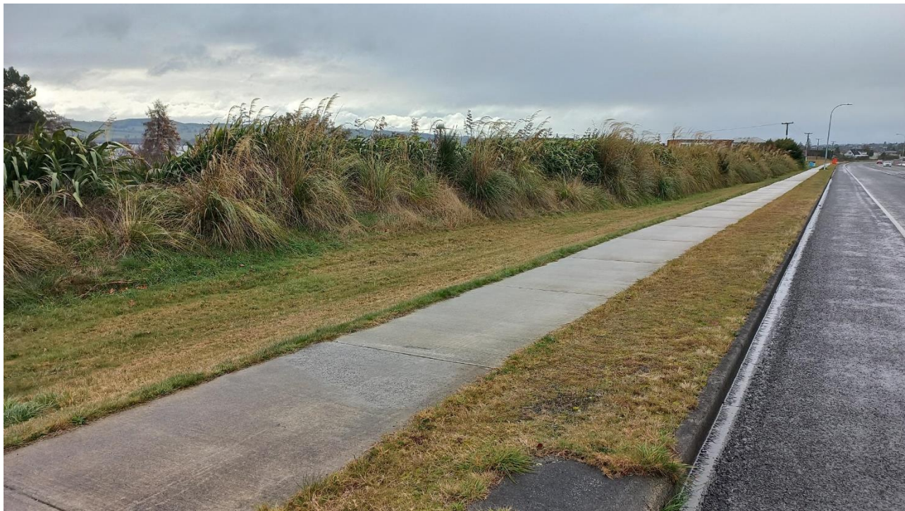
Image 6 – the planted ‘headlight bund’ along Lake Terrace which would no longer be required.
