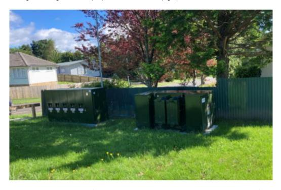
Within each reserve an average 6.0m<sup>2</sup> easement area will be needed: this allows for a 2.1m<sup>2</sup> ring main unit and a 3.0m<sup>2</sup> transformer, separated by a 1.0m gap.
