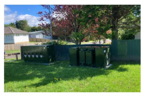
Within each reserve an average  $6.0m^2$  easement area will be needed: this allows for a  $2.1m^2$  ring main unit and a  $3.0m^2$  transformer, separated by a 1.0m gap.
