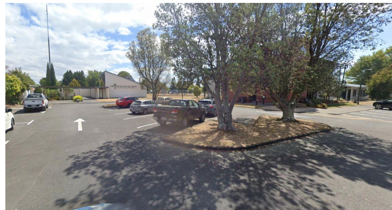
New proposed location of Transformer and Tesla EV Chargers
