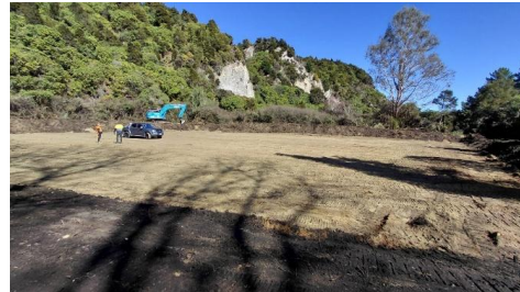
Hatepe Water Treatment Plant Earthworks
