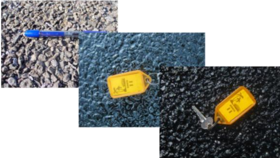
Figure 21 Aitutaki airport bituminous surface preservation treatment 2010
