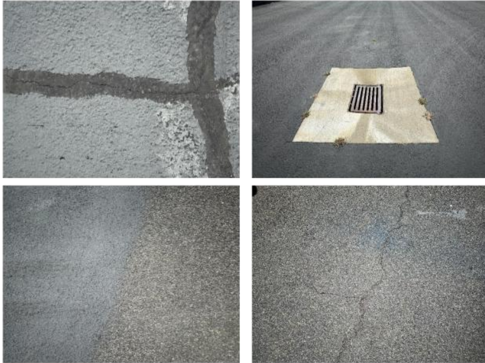
Figure 3-16: GA Apron: Asphalt
