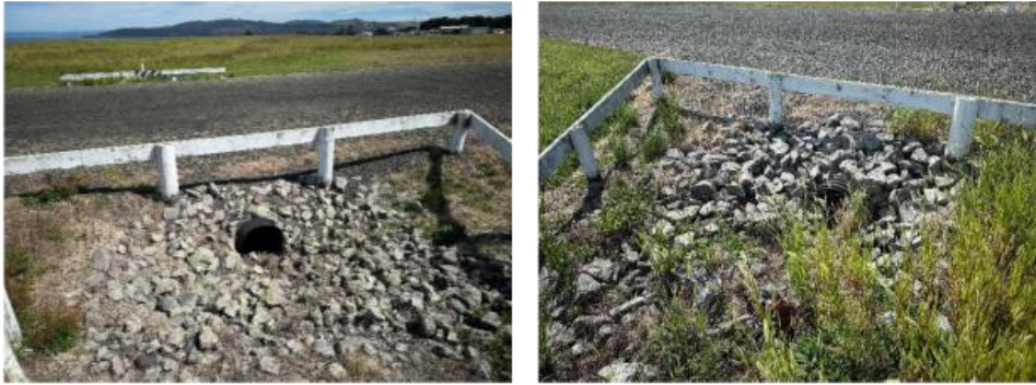
Figure 3-14: Taxiway E – Culvert
